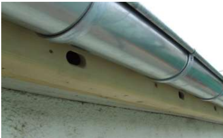
A simple timber box, with internal partitions, that has been fitted under and behind the gutter to form a continuous array of Swift nest places. The entrance holes are sized to resist access by Starlings.
