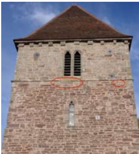
Fig 1: Red circles indicate some of the swift nest sites retained after Repointing works in 2021.
