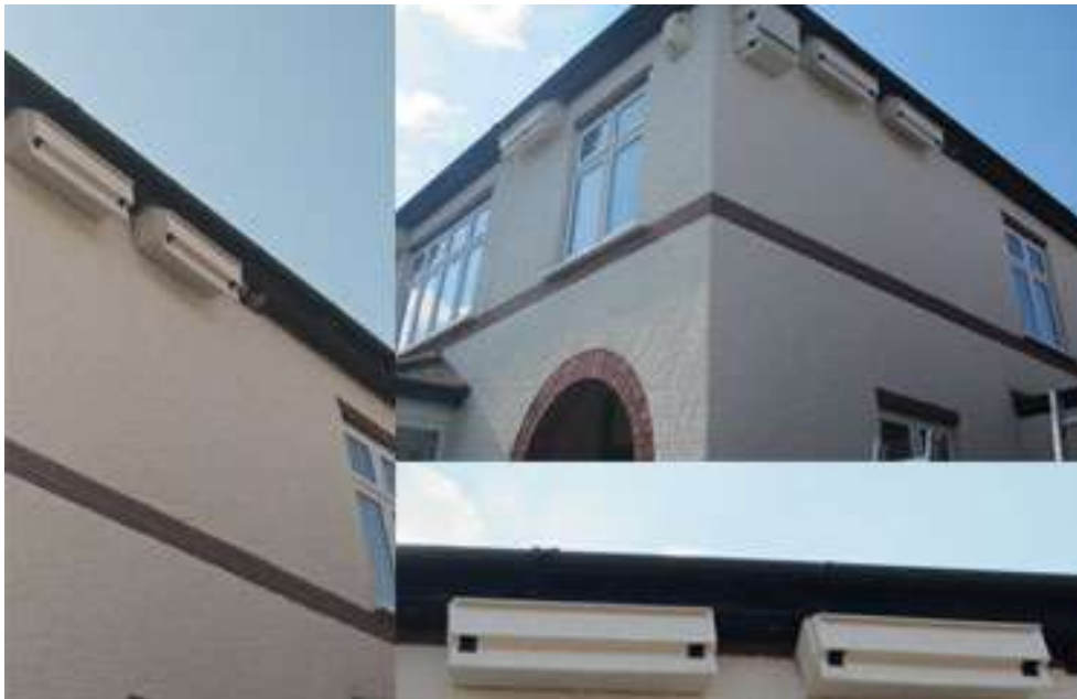
Photos showing finished boxes in position
