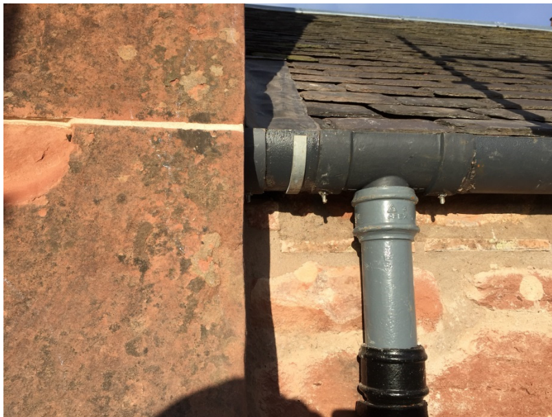
Figure 14 – swift nest site at Inchturre church after renovation © Liz Kay
