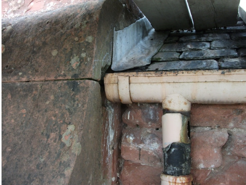
Figure 13 – swift nest site at Inchturre church prior to renovation © Danièle Muir
